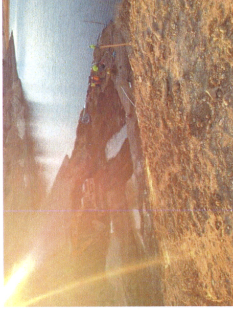
Looking down on the end of the newly installed 20 foot section of pipe. The trench remains flooded with multiple pumps working. Later in the day, about half the trench will be back filled with concrete, capping both culvert sections and joint.
