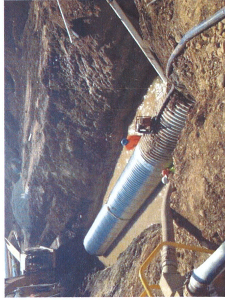
Looking down on the end of the newly installed 20 foot section of pipe. The trench remains flooded with multiple pumps working. Later in the day, about half the trench will be back filled with concrete, capping both culvert sections and joint.
