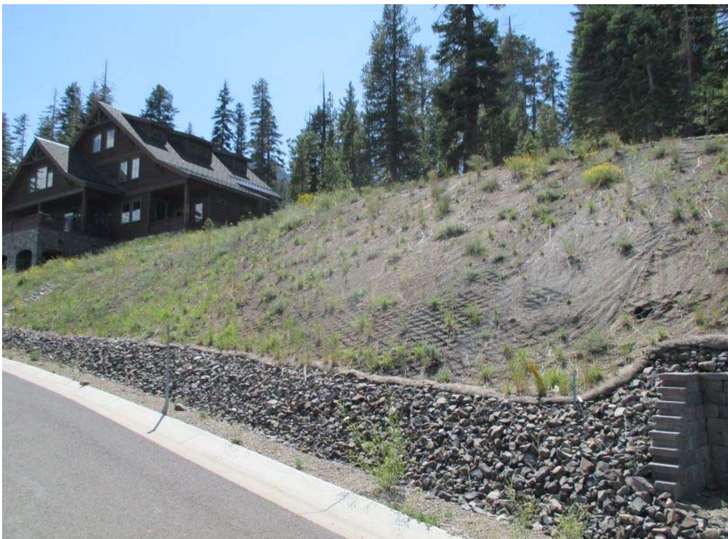
Photo 8. Temporary slope stabilization within Palisades 5. Success of temporary revegetation is variable, but over slope stability maintained by erosion control fabrics and rock as evidenced by lack of dirt and debris on road.
