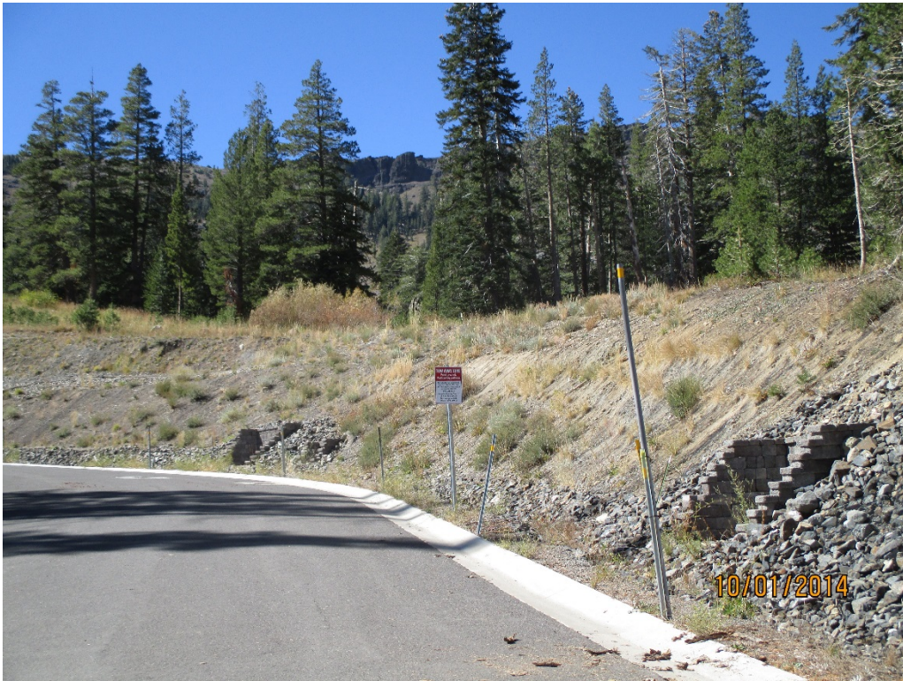
Photo 9. Temporary slope stabilization within Palisades 5. Success of temporary revegetation is variable, but over slope stability maintained by erosion control fabrics and rock as evidenced by lack of dirt and debris on road.
