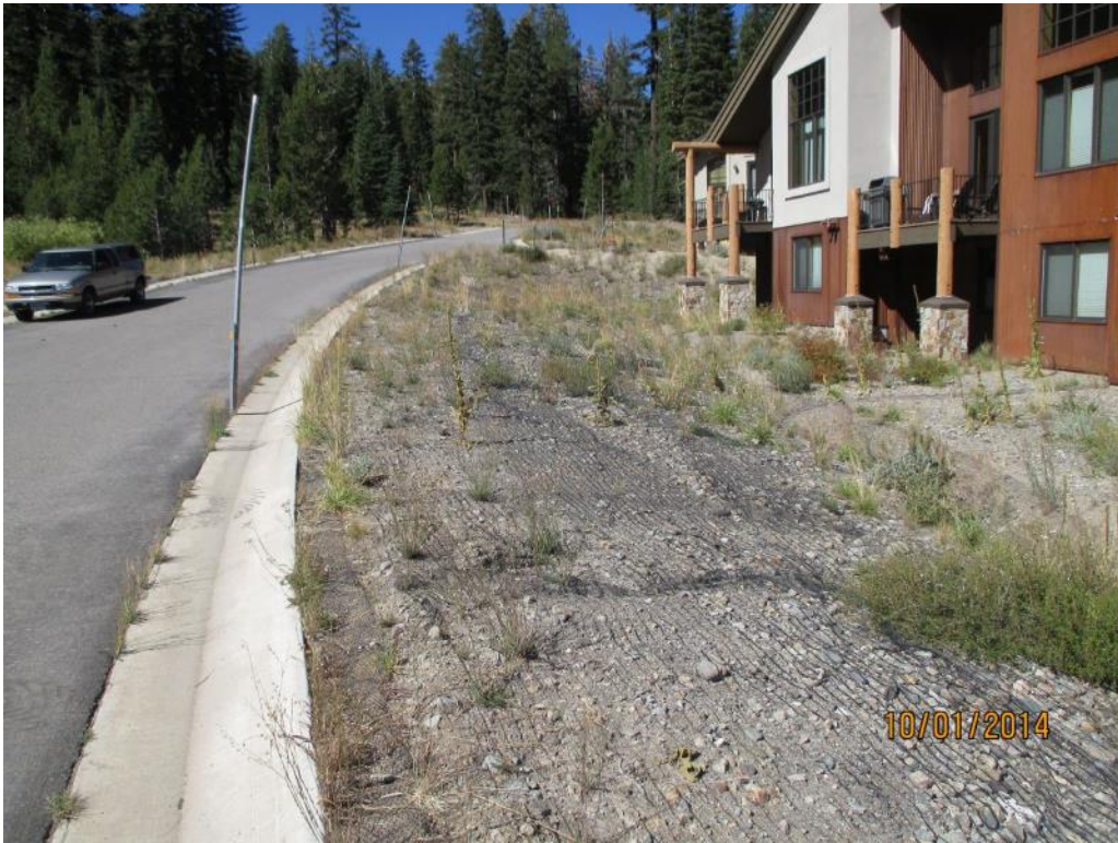
Photo 11. View of failed revegetation along Sentinels Way.
