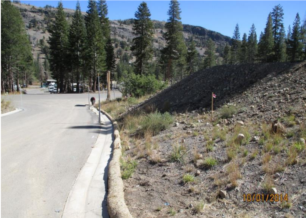
Photo 1. Examples of erosion control material in place during construction of Timber Creek Phase 1.
