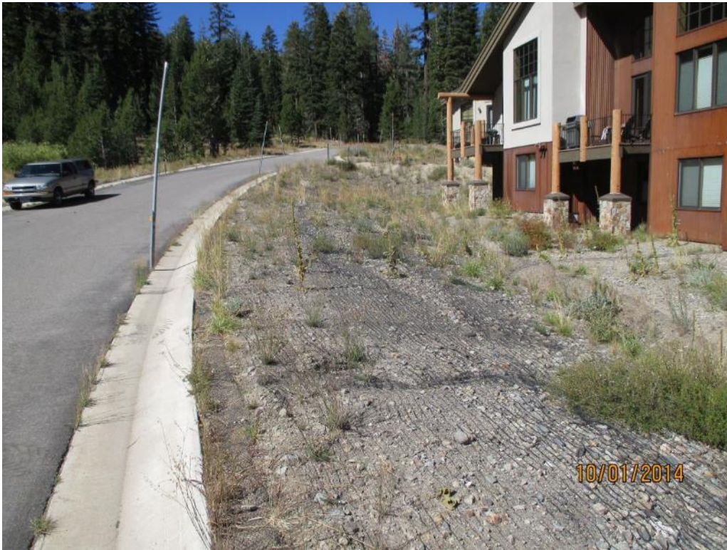
Photo 11. View of failed revegetation along Sentinels Way.
