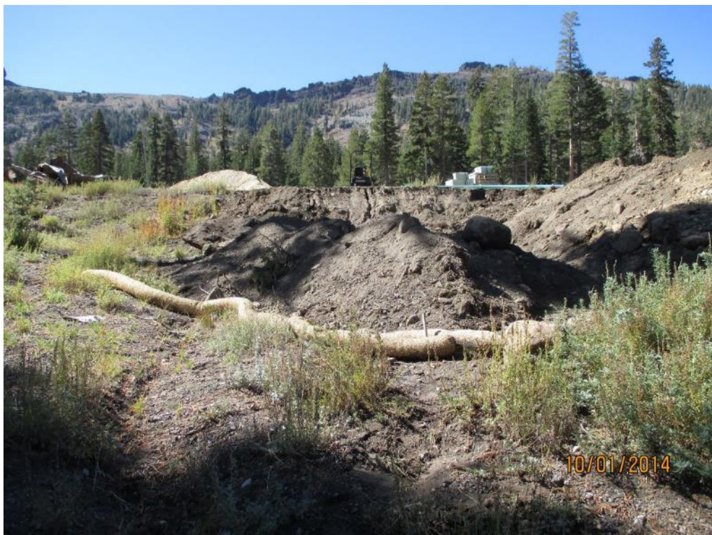
Photo 2. Examples of erosion control material in place during construction of Timber Creek Phase 1.
