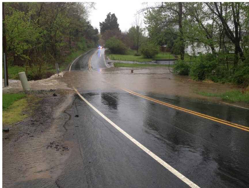
Foothill Type Flooding
