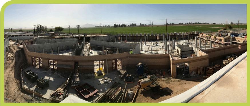
Imperial County Jail Facility Under Construction
