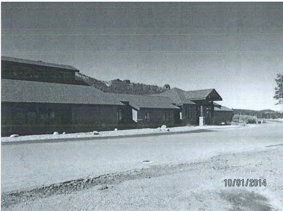
Photo 10. Phase 2 of Kirkwood Recreation Center.
