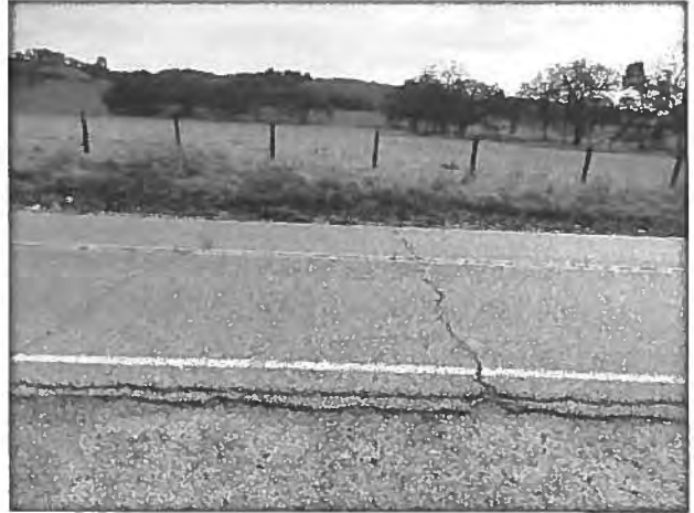
Figure 12- Worn Pavement/Striping on Jackson Valley Road
