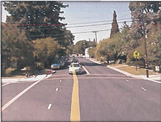
Figure x-Pedestrian Crossing near lone Elementary School from Google Earth
