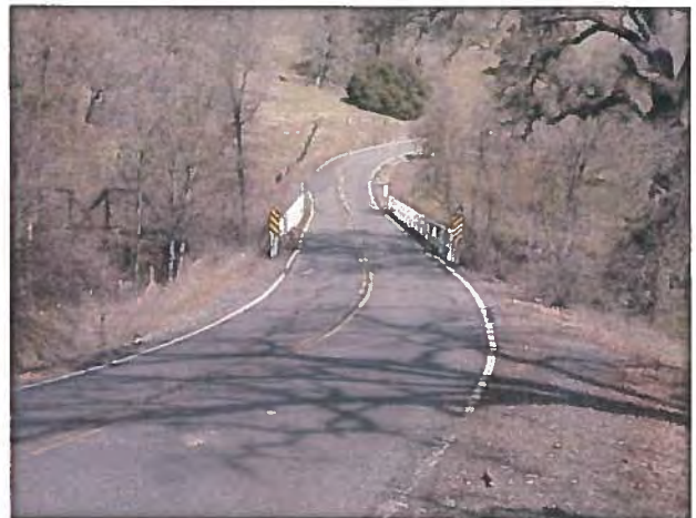
Figure 2- Bridge Crossing Jackson Creek
