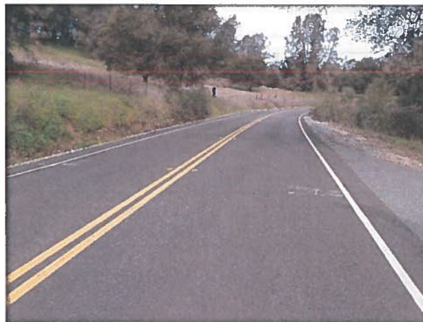
Figure 10- Latrobe Road Curve without Signage
