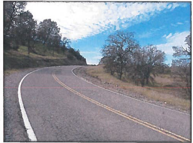
Figure 8- Coal Mine Road Curve without Signage
