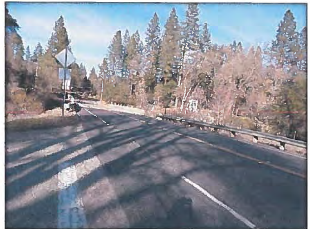
Figure 14- Bridge Crossing Cosumnes River
