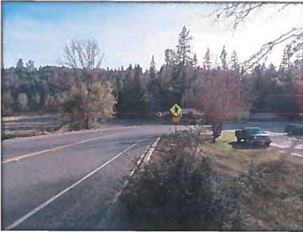
Figure 13- Shenandoah Road Curve with Proper Signage
