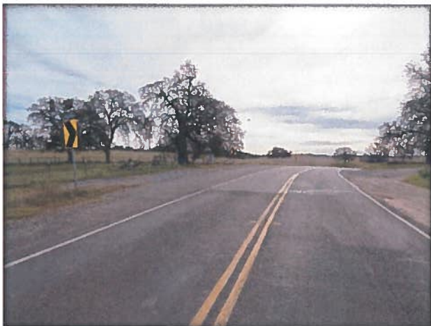
Figure 9- Latrobe Road Curve with Signage
