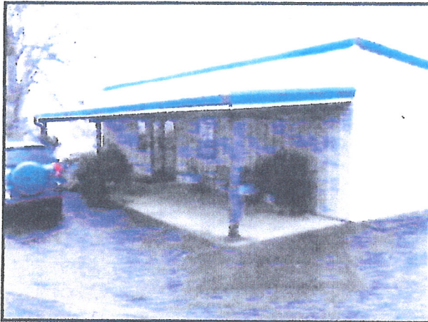
View of veterinary clinic (Building C)
