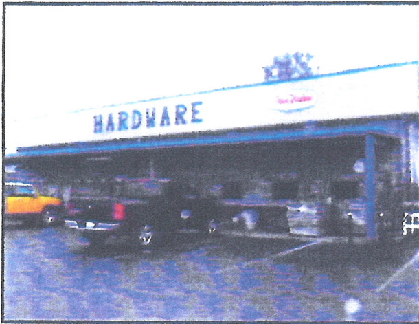
View of hardware store (Building A)
