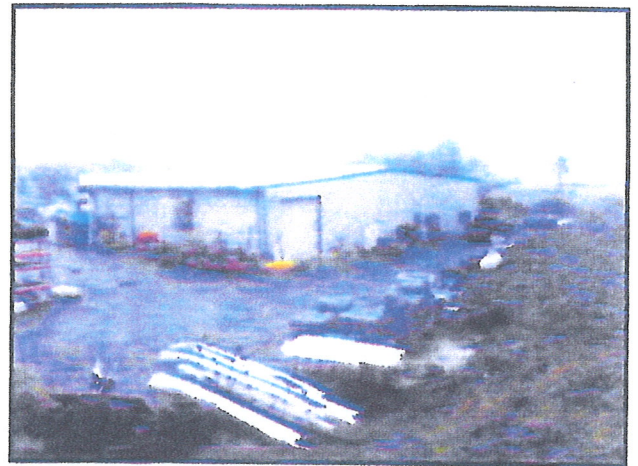
Rear view of hardware store from vet building
