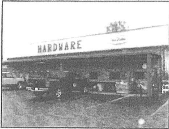
View of hardware store (Building A)
