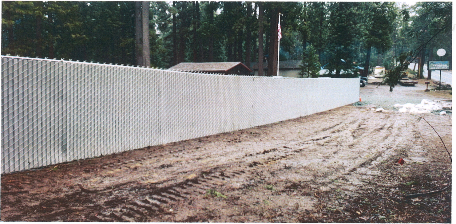
Highway View of Storage Space
