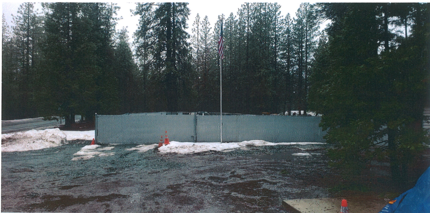
Front view of secured storage space
