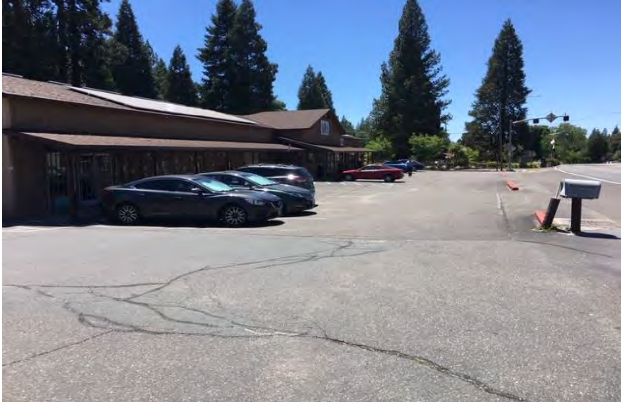
Photo 7: Project area along the frontage with SR 88 to the right. Photo looking west from the northeastern corner of the Project area.
