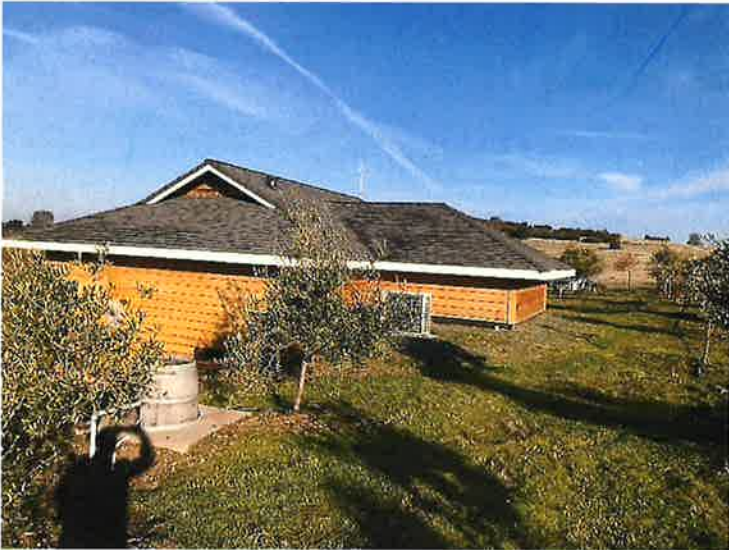
Overview of Project Area showing newly constructed tasting room.
