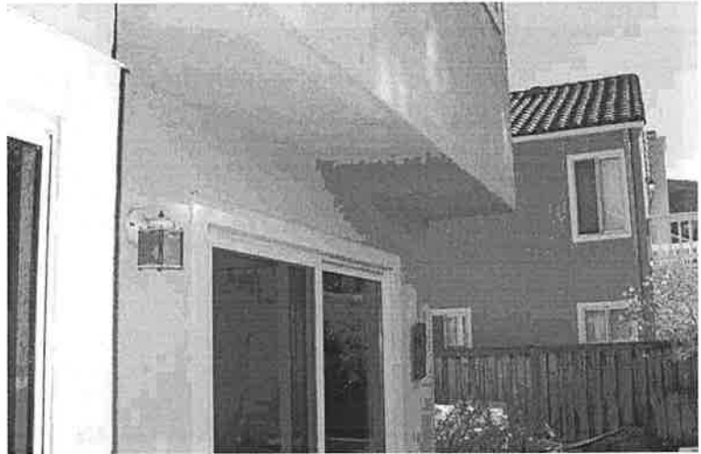
A common house light with no shielding
