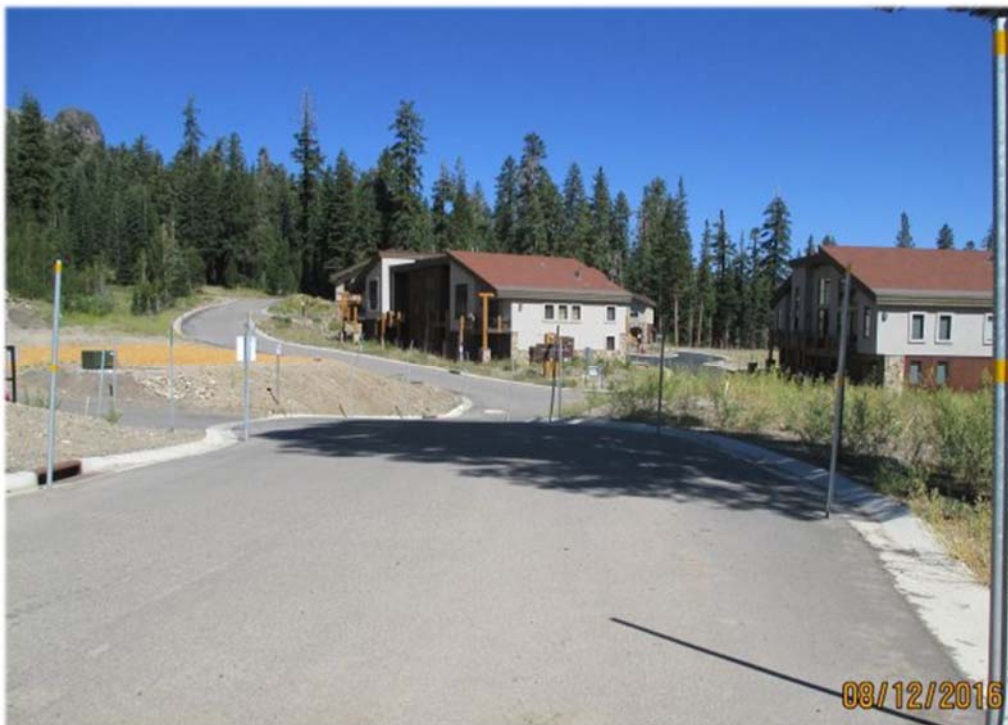
Photo 6. Extension of Sentinels Way Road and development of residential units Sentinel West, located along eastern edge of Martin Point boundary.
