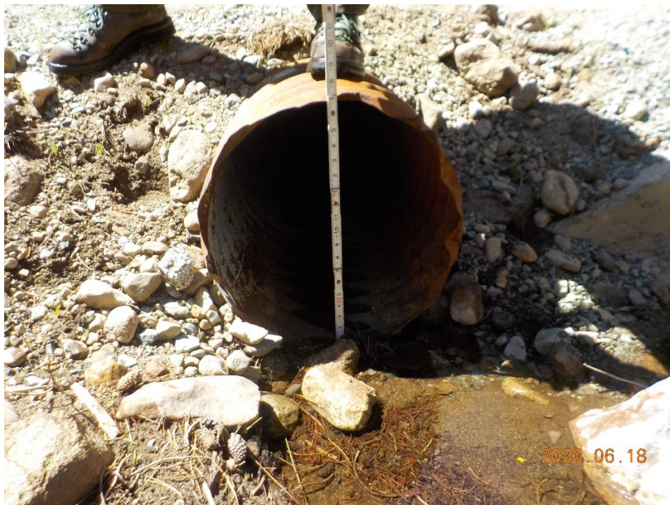
Photo 6. Inlet of 18-inch diameter CMP culvert backfilled with compacted soil and crushed gravel; photo direction – south; June 18, 2020.
