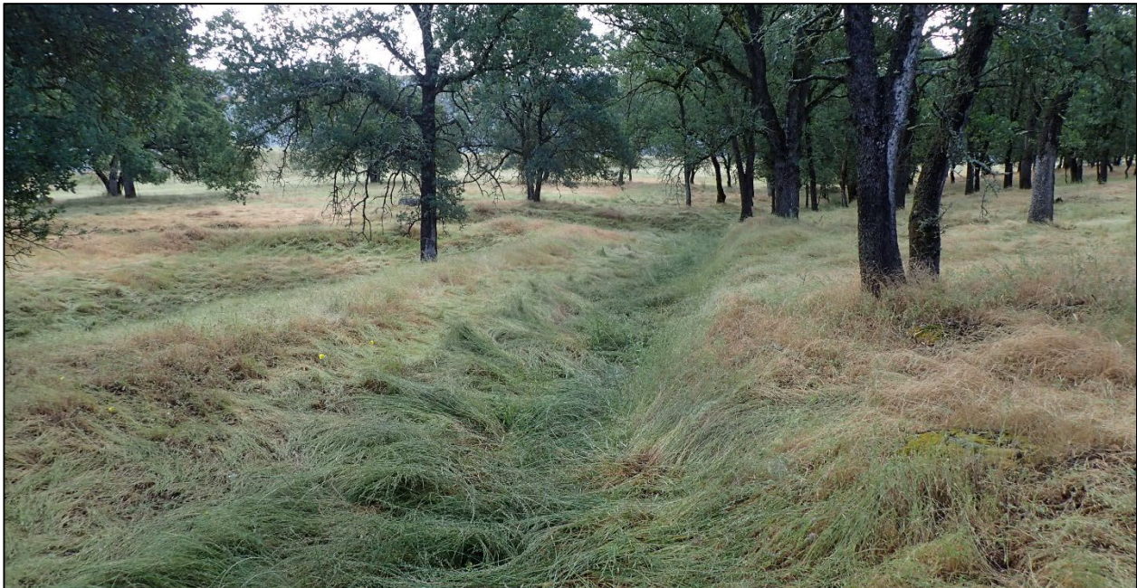
Photograph 6. Non-jurisdictional mining-related drainage ditch located in the southwest portion of the Study Area. This feature terminates in a non-jurisdictional detention basin. Photograph taken May 16, 2019.
