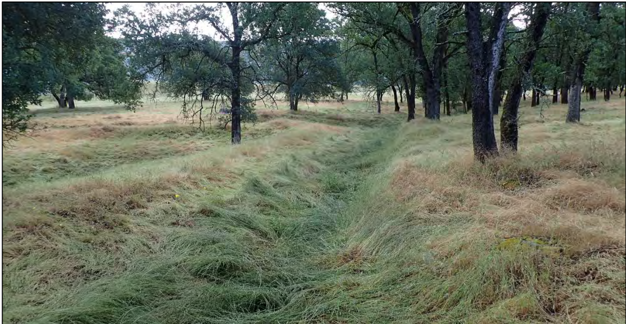
Photograph 8. Non-jurisdictional mining-related drainage ditch located in the southwest portion of the Study Area. This feature terminates in a non-jurisdictional detention basin. Photograph taken May 16, 2019.
