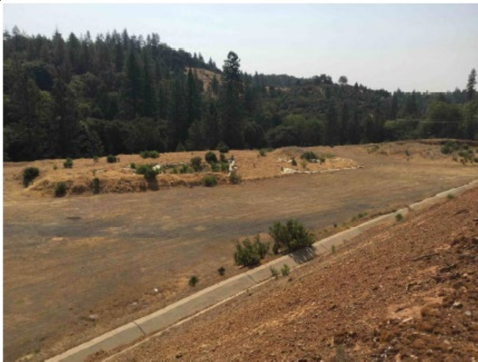
Figure 9-3 Representative photo, looking southeast. Photo taken 9/3/21
