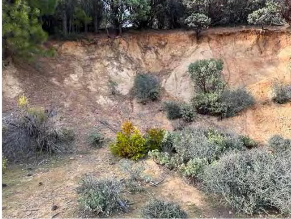
1. View looking north at the cutbank above the project site.
