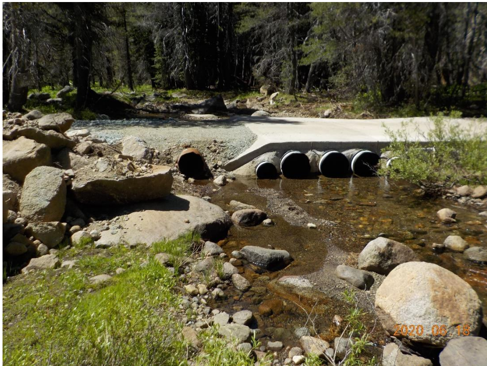
Photo 2. Overview of the constructed crossing with three 18-inch HDPE culverts, two 12-inch HDPE culverts, and one 18-inch CMP culvert; photo direction – south; June 18, 2020.
