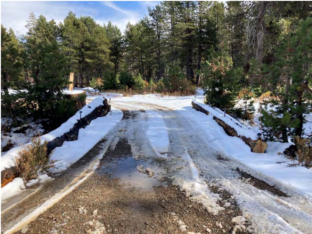
Photo 2. Road and bridge over western stream, facing east (10/19/21)
