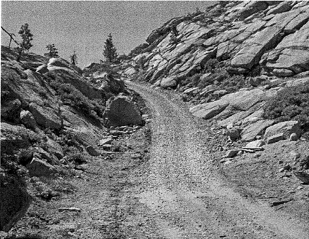
Photo: Road in trespass on Federal parcel.
