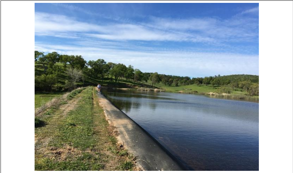
View of the agricultural pond and dam with new liner circa 2010. Source: Lisa Putnam
