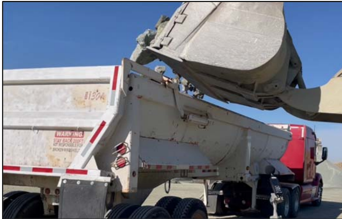
Figure 15 – Loadout of Rip-Rap
