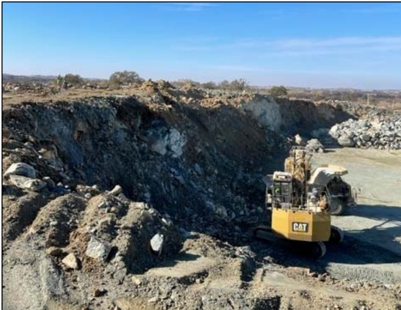
Figure 22 – Shielding of Excavation Activities as Viewed from Bench Above Pit Floor
