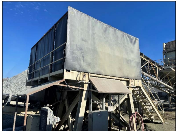
Figure 10 – Crusher GP500 after acoustic curtain installation
