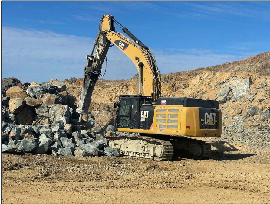
Figure 24 – Excavator-Mounted Pneumatic Rock Breaker
