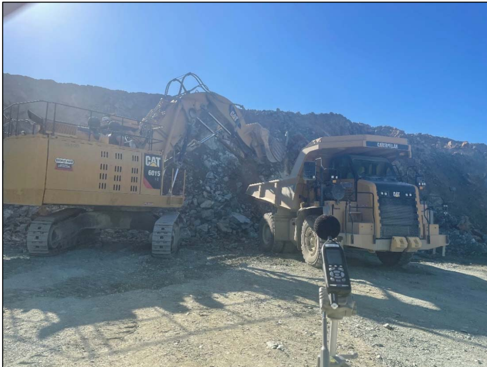
Figure 21 – Unshielded Excavation Activities as Viewed from Pit Floor
