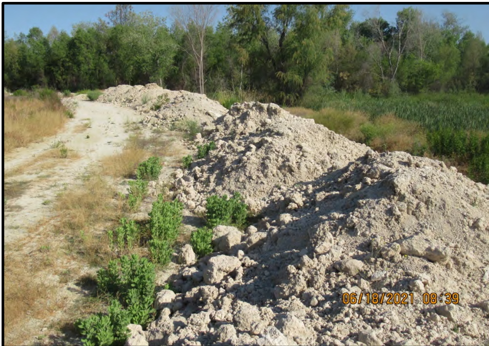
Sediment piles at the west end of the quarry pond, looking northwest; 06/18/21.
