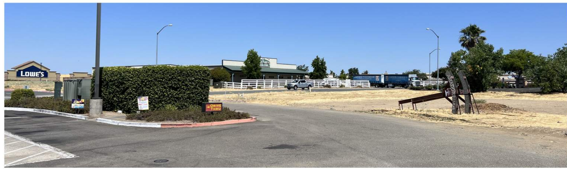
11 SHARED DRIVEWAY LOOKING NORTH TO SITE NOT TO SCALE
